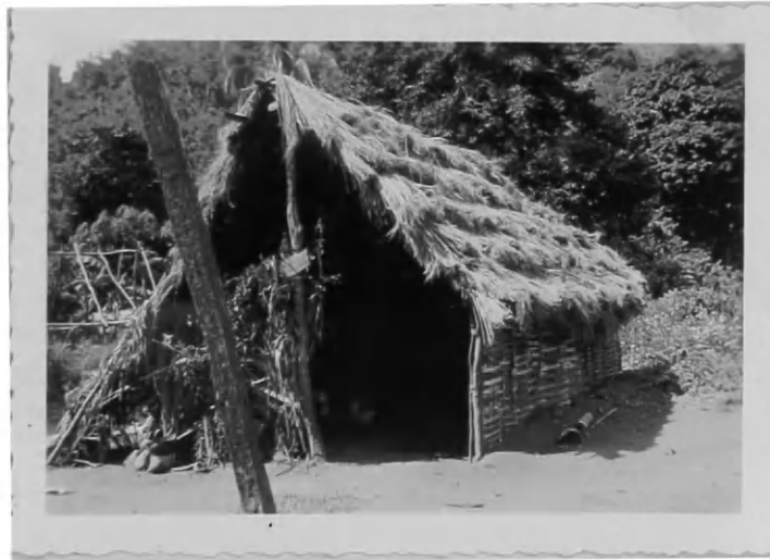
PLATE VII. A ONE-ROOM NATIVE "CAILLE" (DWELLING HOUSE) IN RURAL HAITI, ILLUSTRATIVE OF THE POOREST TYPE OF PEASANT HOMES. (The walls are of plaited palm strips with no adobe, and the roof is of a poor grade of thatch.)
