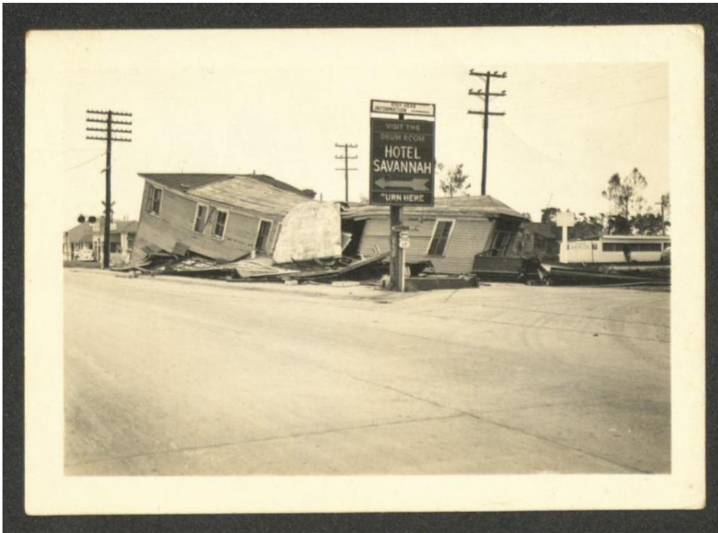
Figure 49. A sign for Hotel Savannah still stands with a building that has been uprooted from its foundation and moved onto the railroad tracks. *Source:* Harr 1940.
