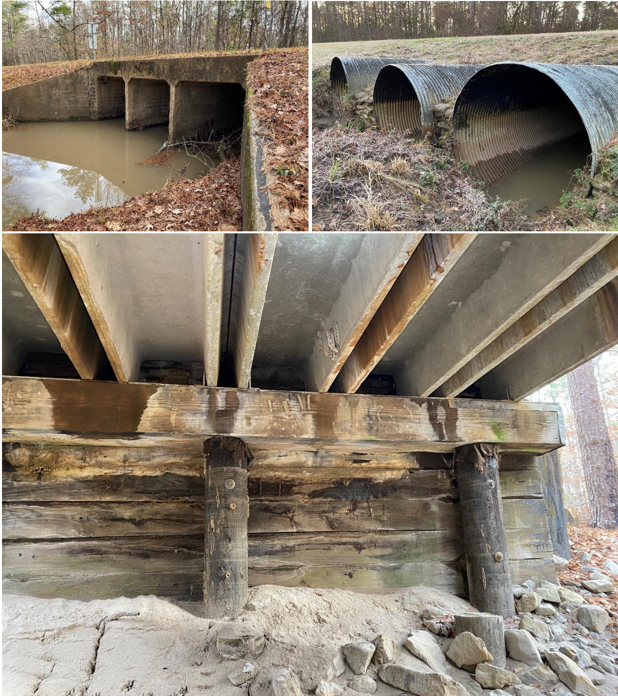
Figure A.1. The three most common structures within 2 km of my study sites, which I found during my study examining the influence of forest management practices on seasonal bat species occurrence and activity in central Louisiana during the non-breeding (January–February 2020 and December 2020–February 2021) and breeding (June–August 2020 and 2021) periods. These structures include box culverts (top-left), circular culverts (top-right), and double-T bridges (bottom).
