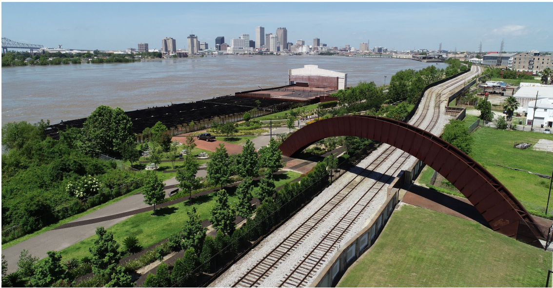
Figure 10. Crescent Park and the steel bridge for pedestrian access to the riverfront park.
