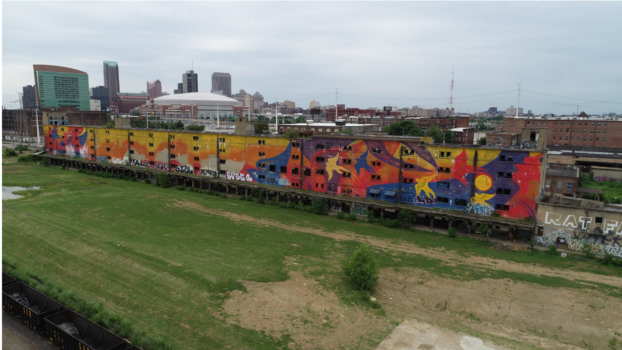
Figure 37. Aerial image at site four, Cotton Belt Freight Depot in Saint Louis, MO.
