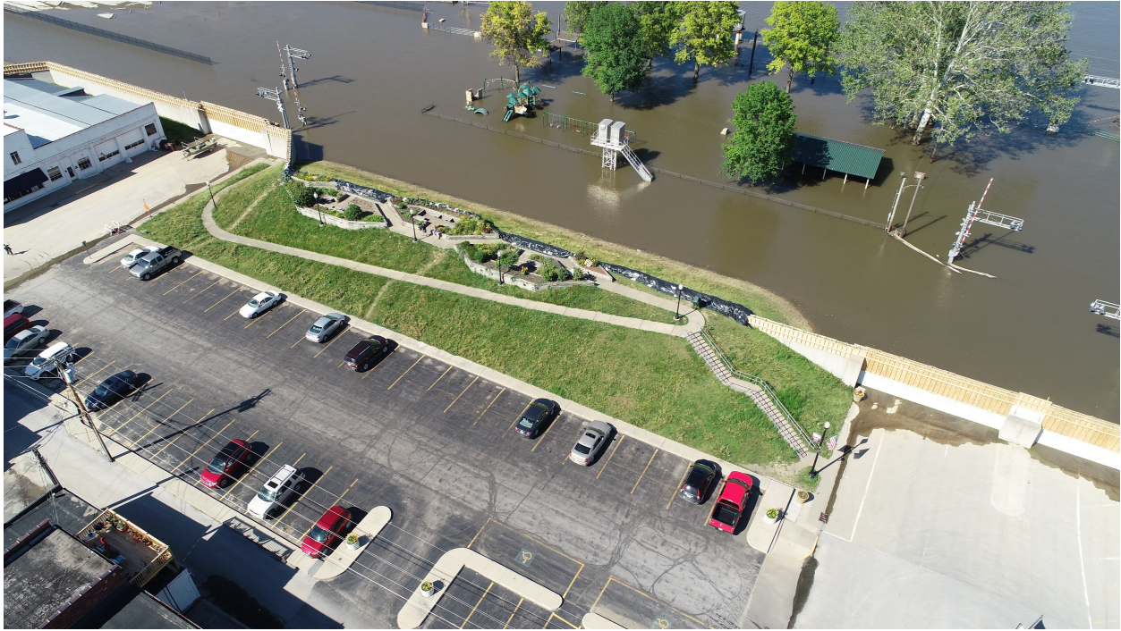
Figure 40. Aerial image of floodwall and levee park on the Mississippi River in Hannibal, MO.
