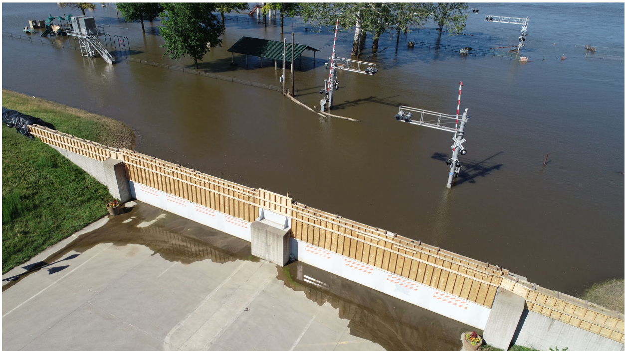
Figure 39. Aerial image of floodwall and the Mississippi River in Hannibal, MO.
