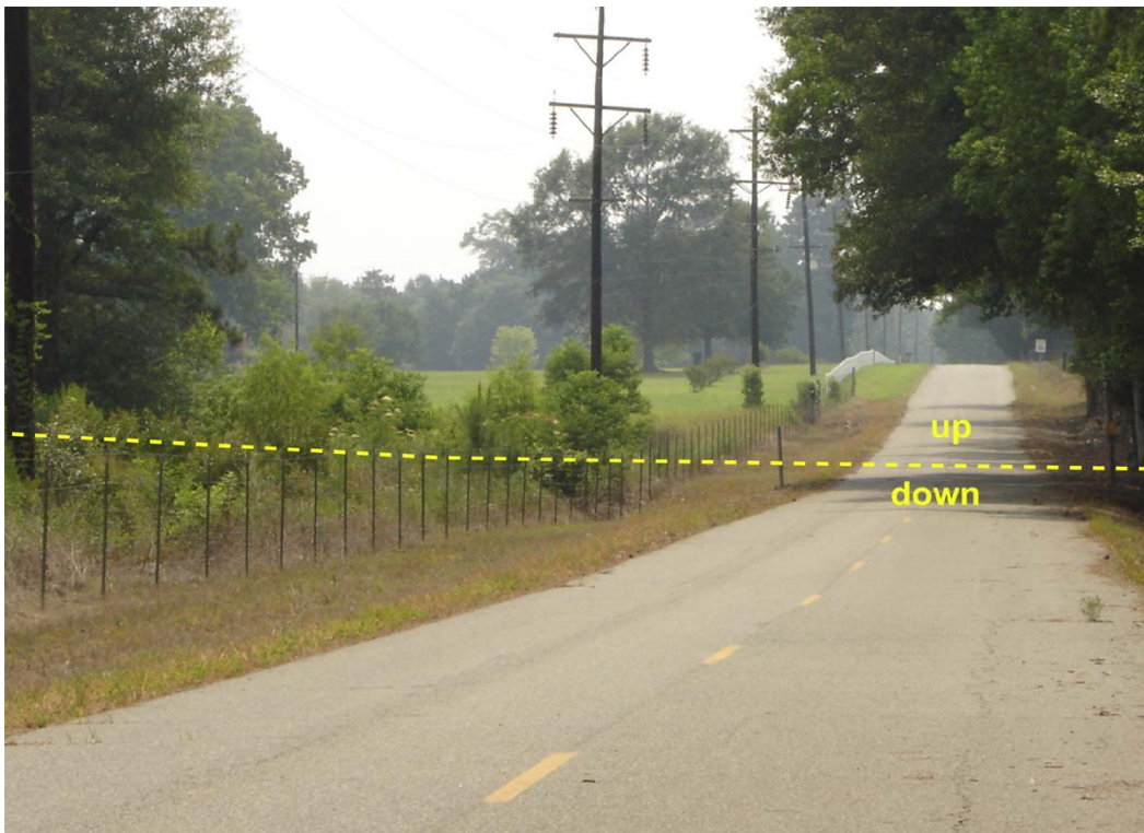
Figure C.6. Photo of the DeQuincy fault-related step near Perkins. The dashed line represents the approximate location of the fault trace.
