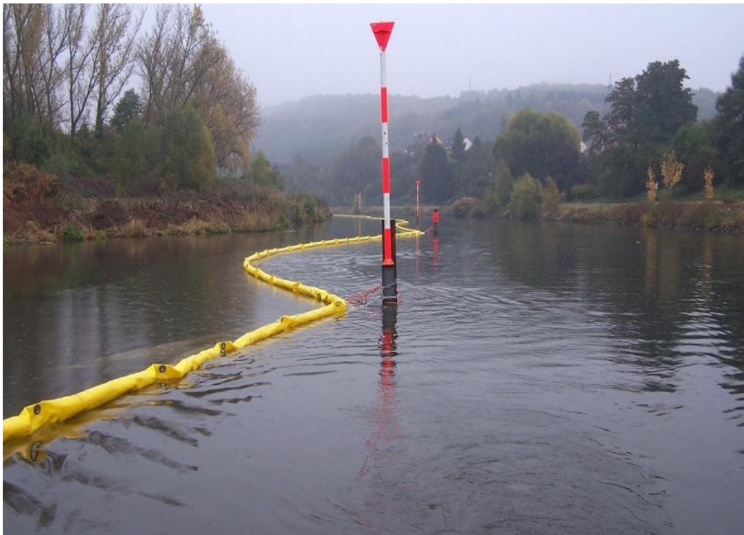
Figure 26 An example of booms which could be used to contain water hyacinth at the shoreline of coastal canals for harvesting and growth (Hydrotechnik, 2012)
