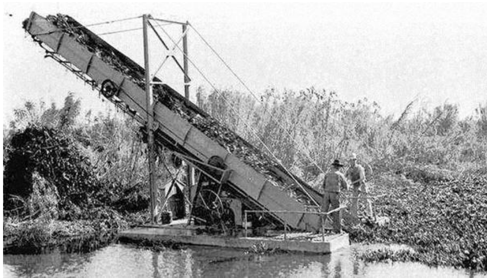
Figure 32 Water Hyacinth Mechanical Elevator Barge from the early 1900's, unknown photographer (University of Florida IFAS Extension, 2012)
