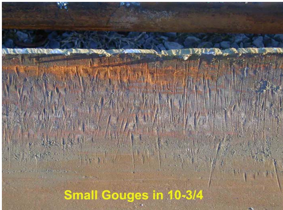
Figure 5-3: Slight Scarring of 10 3/4-in. Casing from Milling Operation
