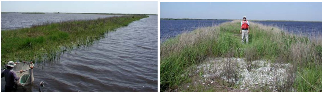
Figure 3. Unit 7 terraces built in 1999.
