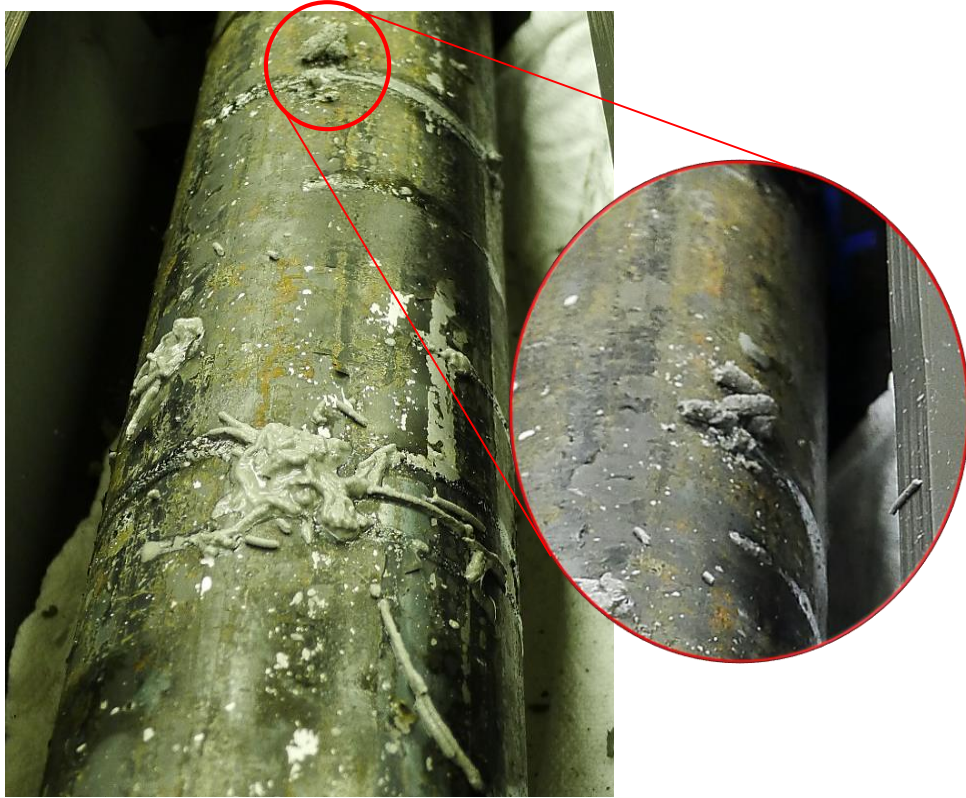
Figure 4.1: Photo of a composite sample after expansion with the 8% expansion ratio cone. Fully hydrated cement, with a paste-like consistency, has been squeezed out from the holes on the outer pipe together with free cement pore water. The magnified view showing cement paste squeezed out from larger holes.
