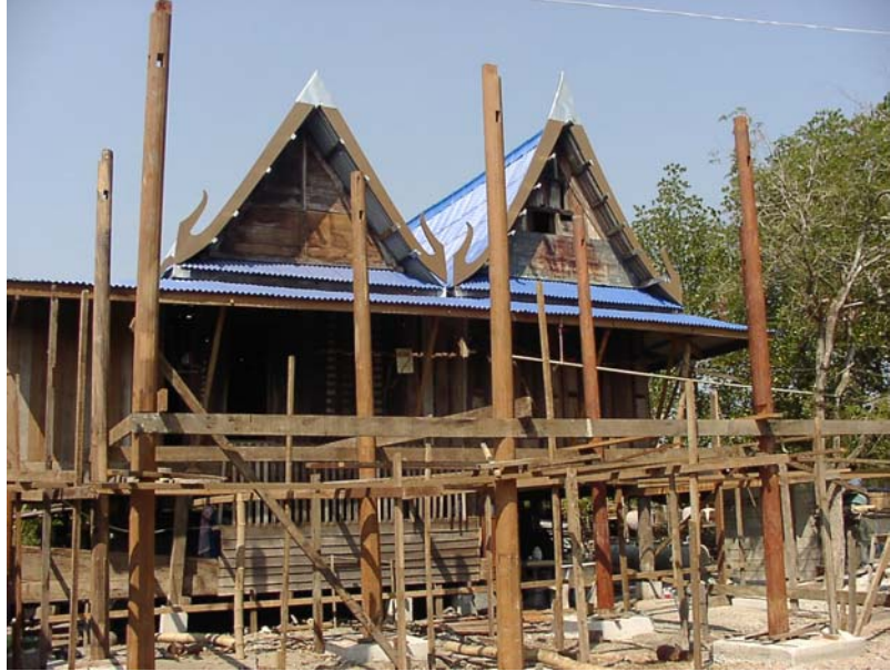
Figure 27. Local people's house (under construction)
