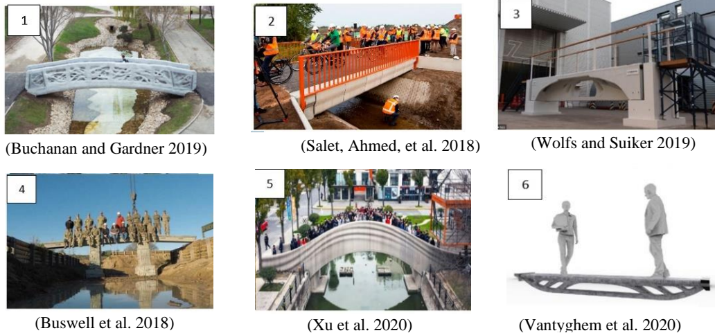
Figure 3. Application of 3DCP in pedestrian bridge construction
