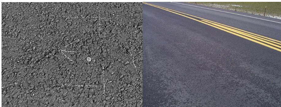
Figure 1. Aggregate Segregation and Non-Uniform Texture after Construction (3)
