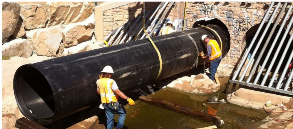
FIGURE 3 Culvert retrofit using HDPE pipes [2].
