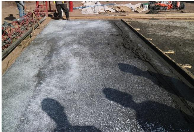
**Figure 16. Mock-up placement 4 – UHPC finish.**
