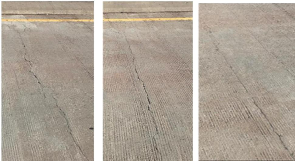
Figure 8. Transverse cracks observed on the concrete bridge deck.
