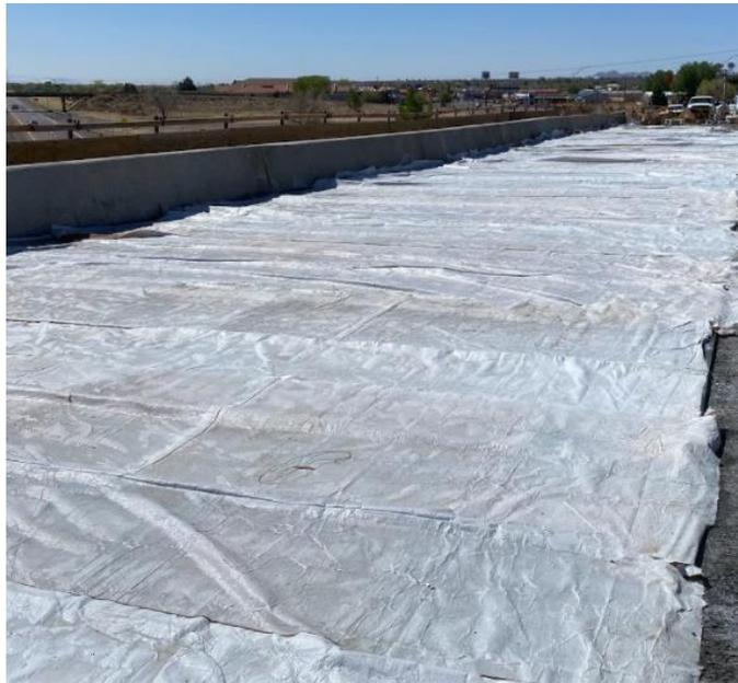
**Figure 42. UHPC overlay covered with plastic sheeting.**
