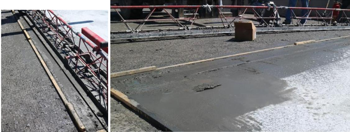
Figure 43. Images of construction joint blocking.
