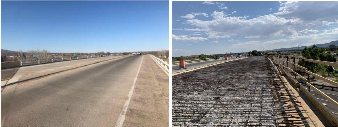
Figure 27. Bridge 7032 before and after first deck section removal.
