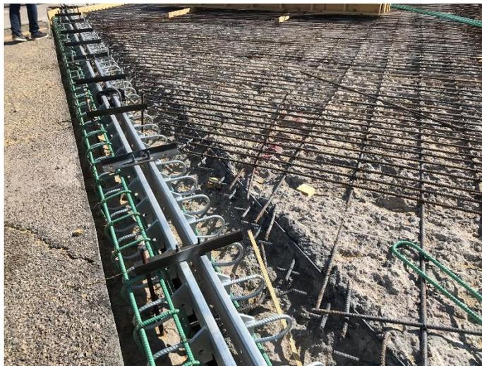
Figure 10. Replacement of the expansion joint seal.
