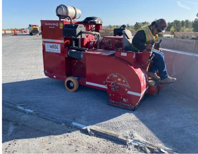
**Figure 25. Ceramic bead blaster.**
