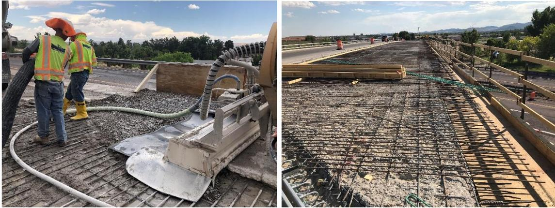
Figure 9. Condition of deck on southbound lane after removal of deteriorated concrete.
