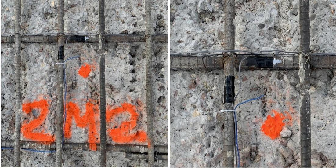
**Figure 29. Embedded sensor installation in HPD.**
