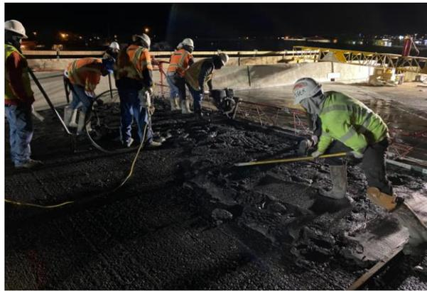
**Figure 39. Construction workers spreading UHPC with shovels prior to screeding.**
