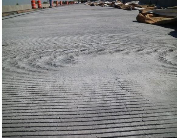
Figure 26. Production placement 1 – UHPC overlay cracking.
