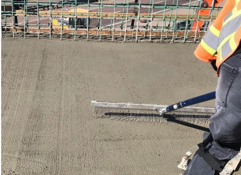
Figure 24. Tine rake used to texture the HPD surface.
