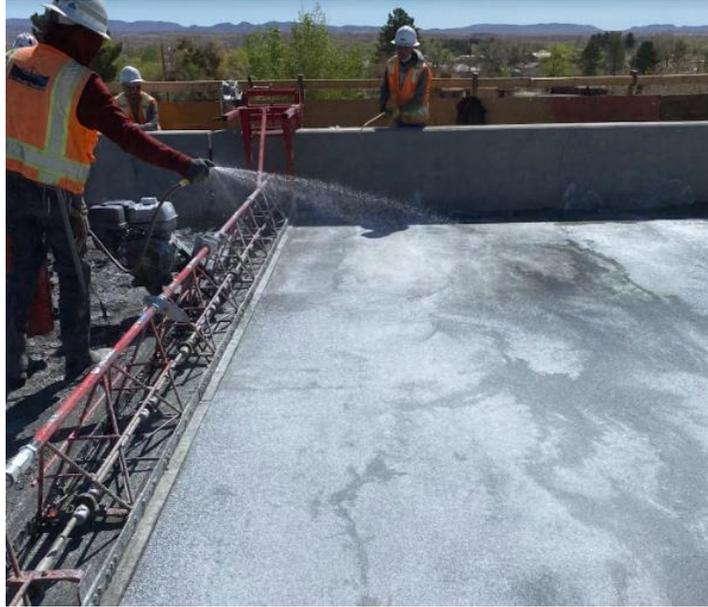
**Figure 41. Application of curing compound after screeding.**
