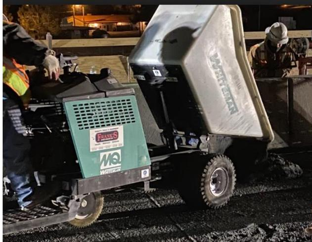
**Figure 38. Concrete buggy delivering UHPC.**
