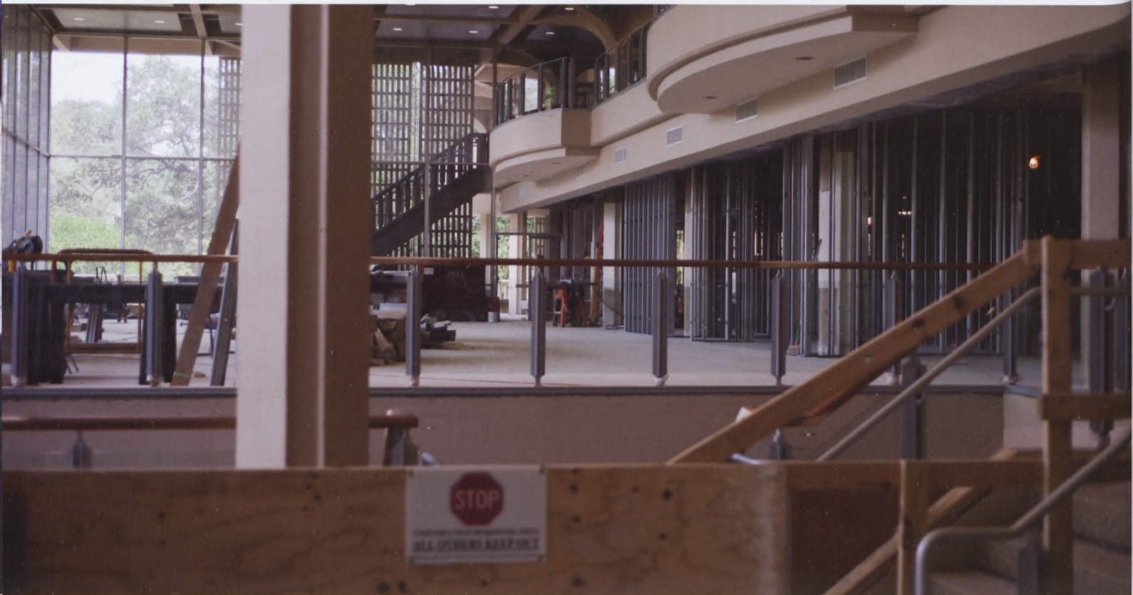
The Union construction is almost finished! | Robert Giglio
