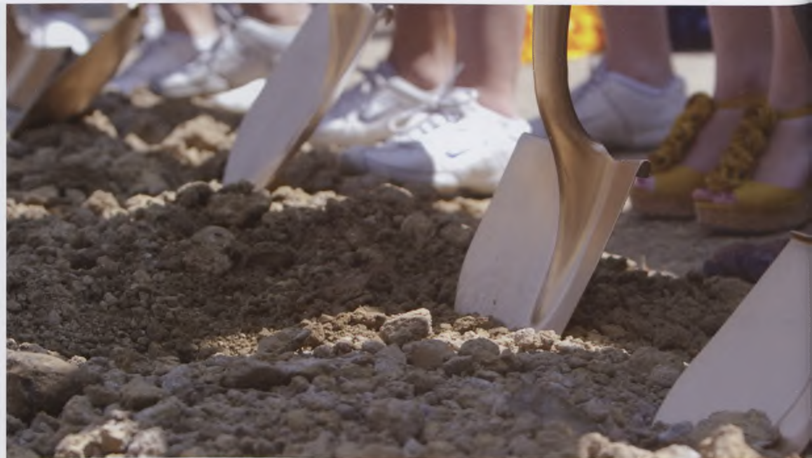
Shiny shovels break the ground for the new complex. | Photos by Martin McCallister
