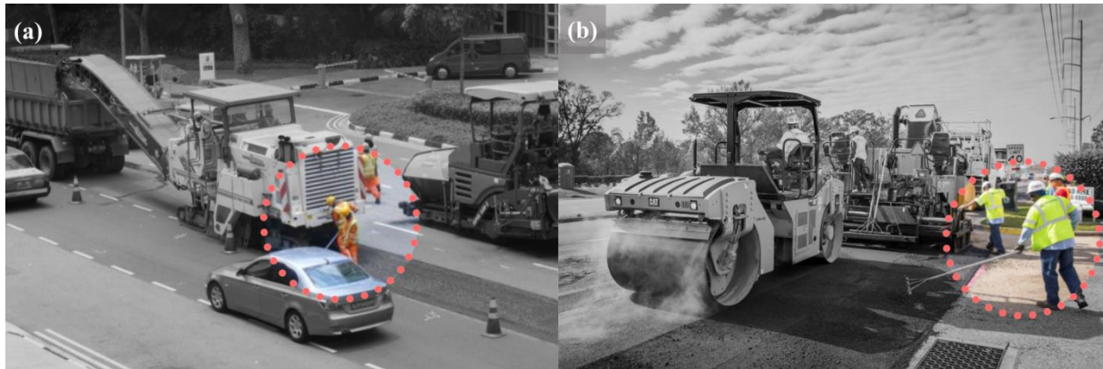
Figure 1. Road construction workers, exposed to multiple struck-by hazards: (a) Workers at an asphalt milling worksite (4), (b) Workers at asphalt paving worksite (5).
