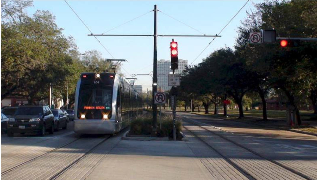
Figure 58. Textured concrete marking of LRV track area, Houston Metro, TX
