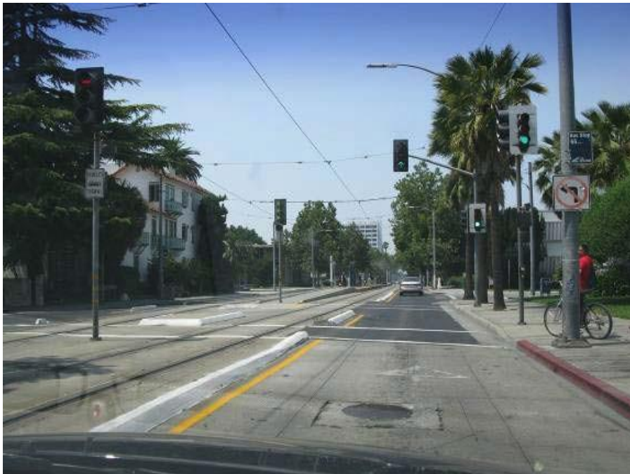
Figure 13. Type b.3 Alignment with Barrier Curbs Santa Clara SCVTA, CA
