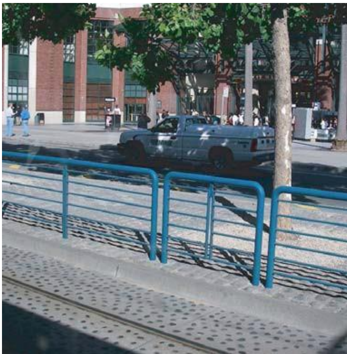
Figure 48. Pedestrian fencing near stadium stop, Muni's T and N lines, San Francisco, CA
