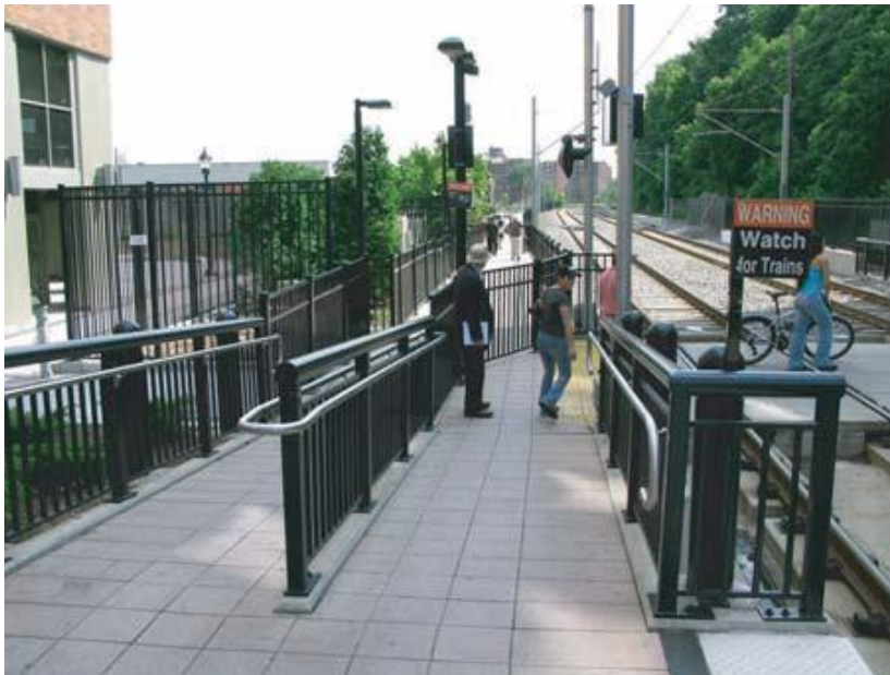
Figure 53. Offset pedestrian crossing at an LRT station Hudson-Bergen Line, NJ
