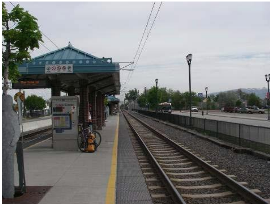
Figure 7. Example of type-a exclusive alignment Salt Lake City, Sandy Line, UT
