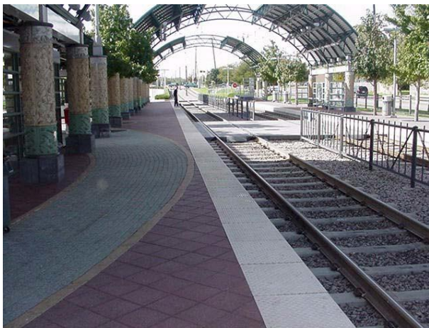
Figure 67. Paint and texture on station platform edges, DART, Dallas, TX
