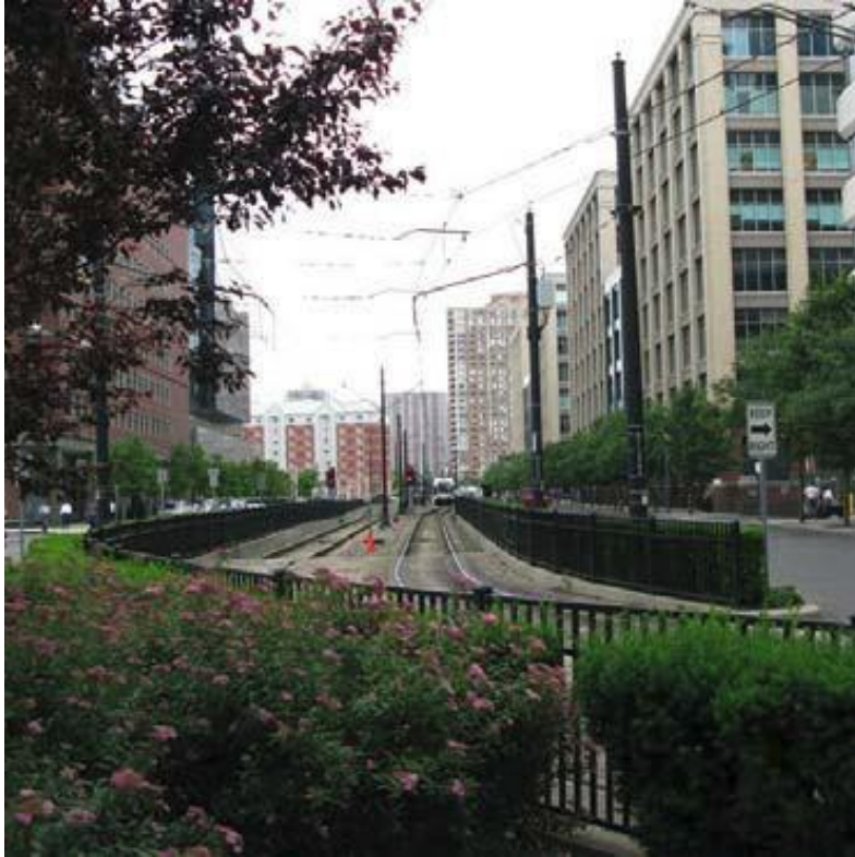
Figure 47. Pedestrian fencing and landscaping in a downtown area with significant pedestrian traffic, Hudson–Bergen LRT, NJ
