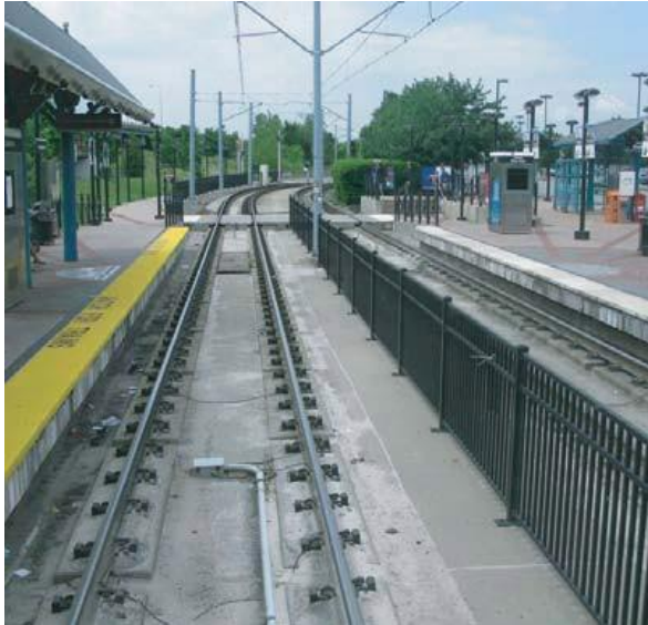
Figure 63. Paint and texture on station platform edges, Hudson-Bergen line, NJ
