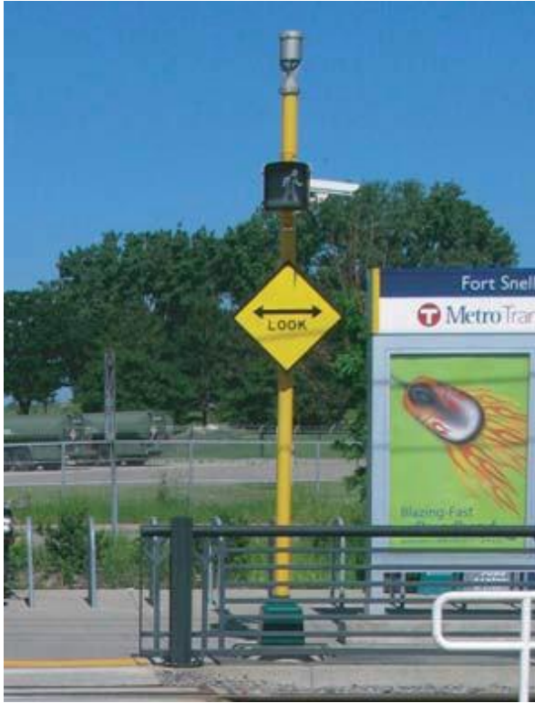
Figure 29. Pedestrian signal with audible crossing warning device and “LOOK BOTH WAYS” sign, Hiawatha line, Minneapolis, MN
