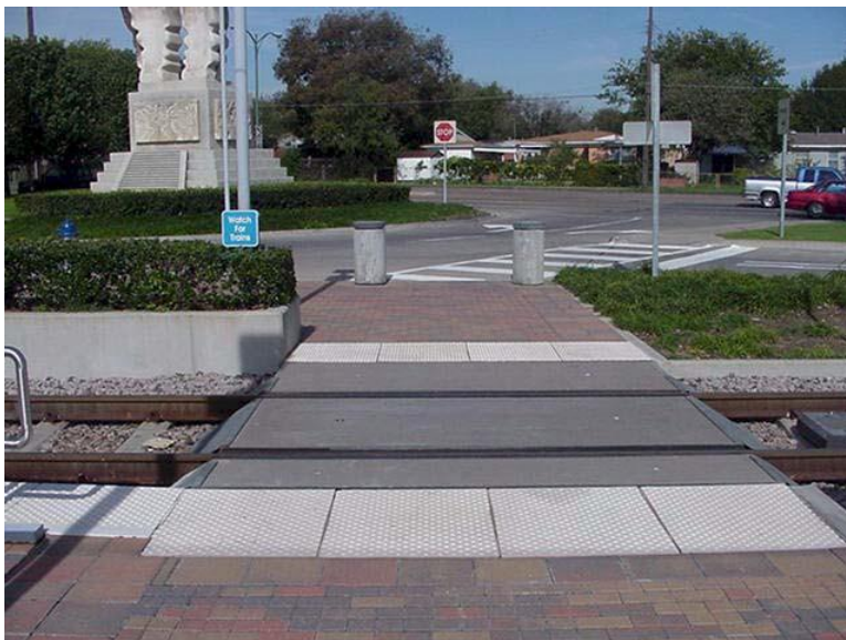
Figure 64. Textured concrete and tactile strips marking the pedestrian crossing area, DART, Dallas, TX
