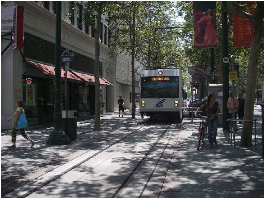
Figure 19. Type c.3 alignment with pedestrian mall Santa Clara SCVTA, CA
