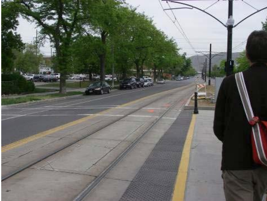
Figure 14. Type b-4 Semi-exclusive Alignment - Rumble Strip and Pavement Markings Salt Lake City, UT
