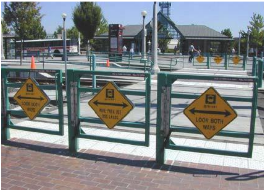
Figure 45. Pedestrian swing gates, Tri-Met LRT, Portland, OR
