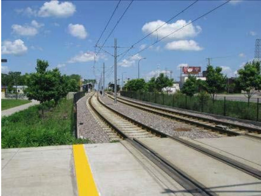
Figure 10. Typical Type b.2 Station Minneapolis Metro Transit, MN
