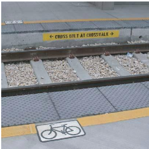
Figure 62. Painted “CROSS ONLY AT CROSSWALK” marking and tactile strips at an LRT station, Salt Lake City, UT
