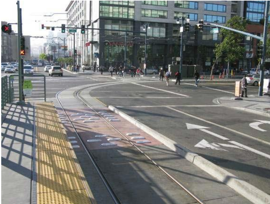
Figure 16. Intersection on Semi-exclusive Alignment San Francisco MUNI, CA
