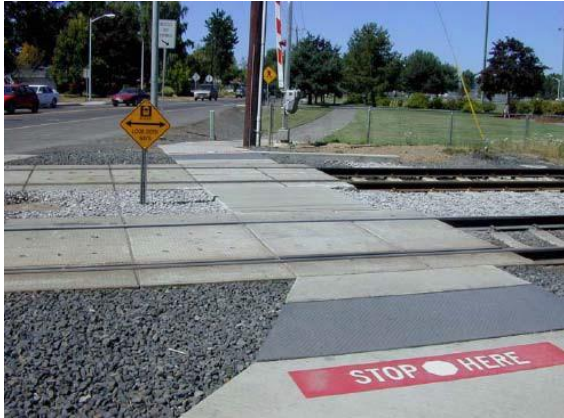
Figure 60. Painted “STOP HERE” on concrete pedestrian path before crossing, Tri-Met, Portland, OR
