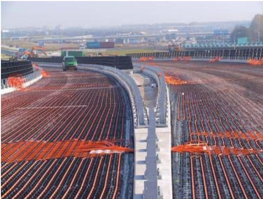
Figure 4. Asphalt solar collector system under construction on a bridge in Rotterdam (14)
