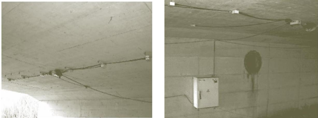
**Figure 22. Slovenia B-WIM Technology (Source: Commercial Motor Vehicle Size and Weight in Europe)**
