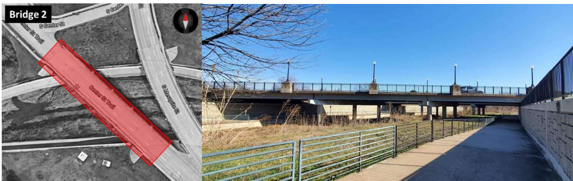
Figure 4. The photo of the second candidate (Bridge 2) on Center St. Trail Arlington
