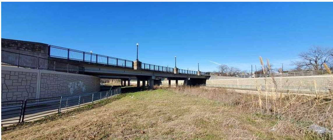
Figure 3. The photo of the first candidate (Bridge 1) on S Mesquite St. Arlington
