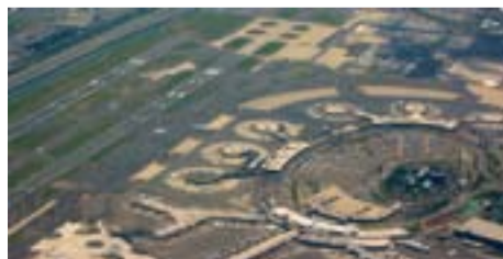
Newark International Airport
