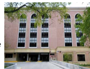
New Parking Garage, Raphael Semmes Road Entrance
