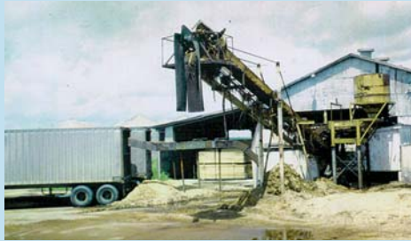
Sawdust, bark and wood trimmings from this hardwood mill are trucked to a paper mill. Some of the material is used to make paper, while the rest is used for energy.
